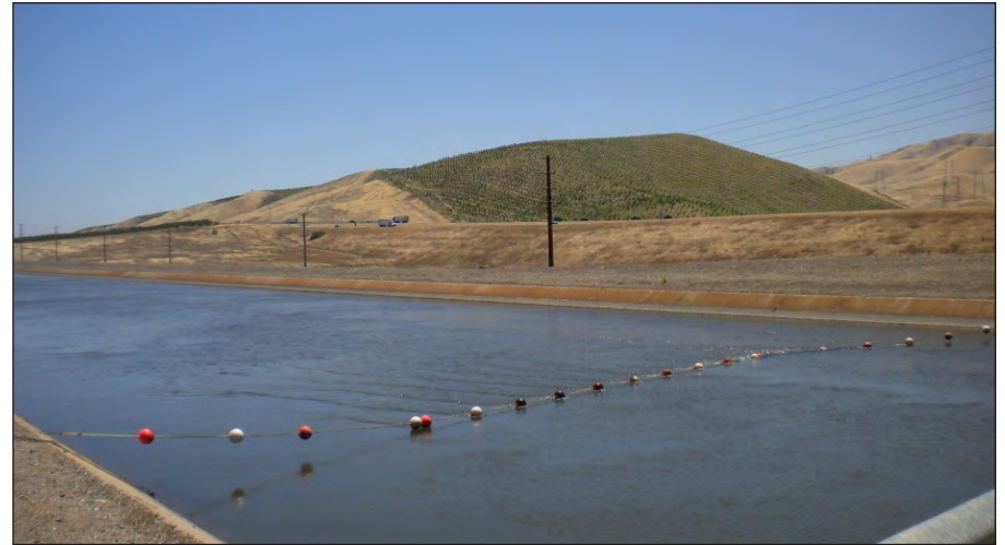
Photograph 2: View of the California Aqueduct looking south.
