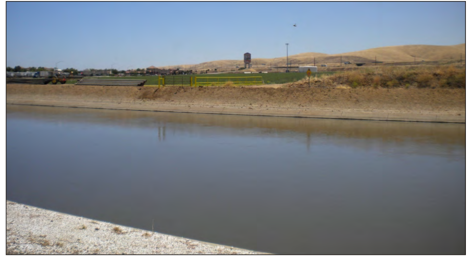
Photograph 2: View of the Delta-Mendota Canal looking south.
