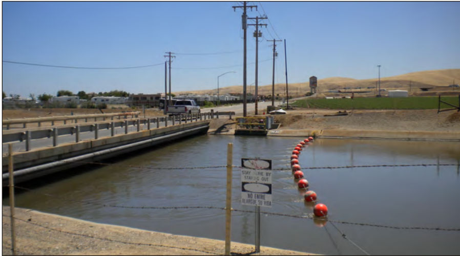
Photograph 3: View of Rogers Road crossing of the Delta-Mendota Canal.
