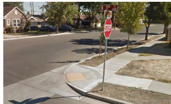
ADA-Compliant Curb Ramp
