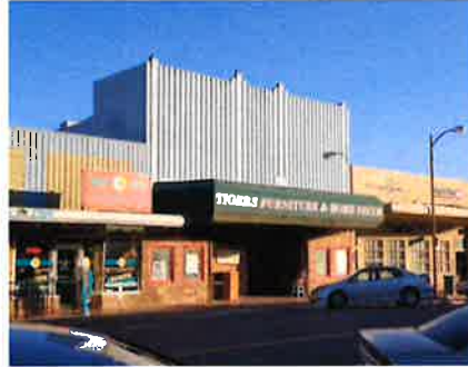
FURNITURE STORE IN OLD THEATER BUILDING
