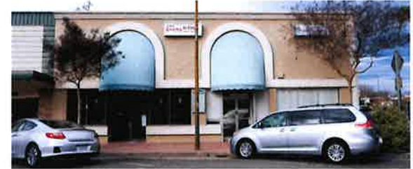
A historic building on S. Del Puerto that was covered with a stucco facade that does not reflect the historic architectural character.
