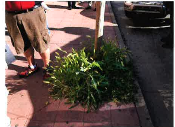
Weeds and cracked sidewalks were seen on S. Del Puerto Avenue.
