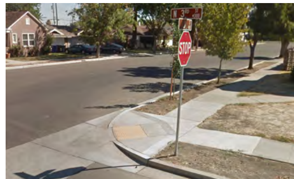
ADA-Compliant Curb Ramp
