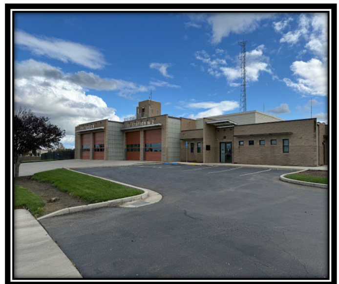
Fire Station # 2 1950 Keystone Pacific Pkwy.
